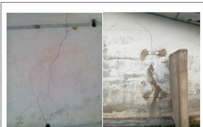
Figure 1: Walls cracked.
