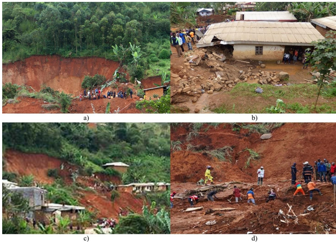
Figure 2: Recent landslides in the West Region of Cameroon, (a) Landslide scar. (b) demolished house along landslide path. (c) constructed houses along unstable slope. (d) recovery of materials and human remains from landslide debris.
